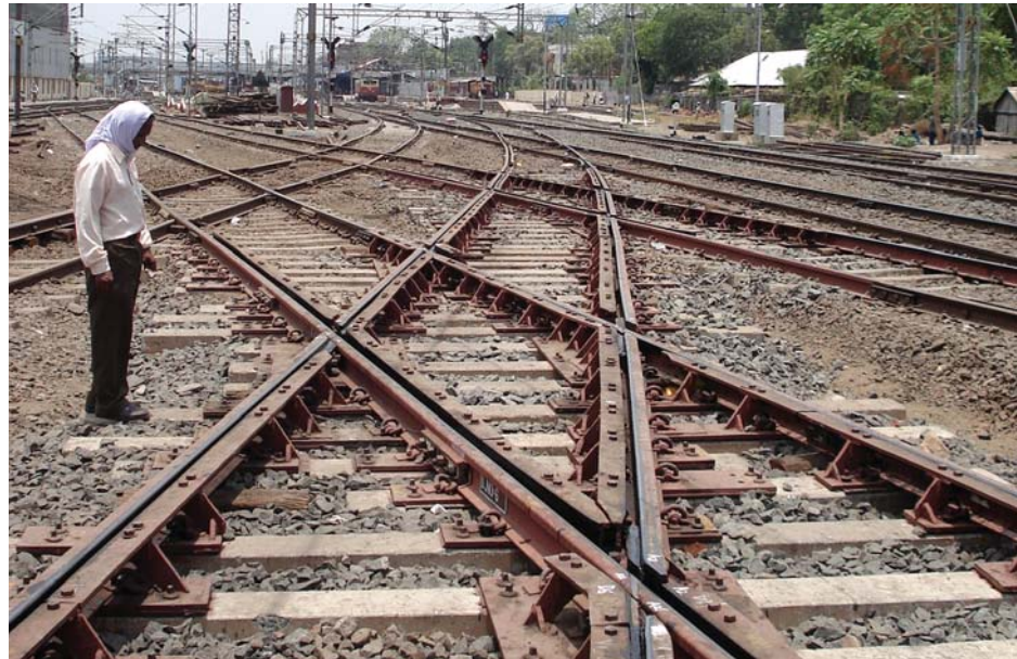
Experimental diamond assembly on concrete sleepers at Bhusaval
