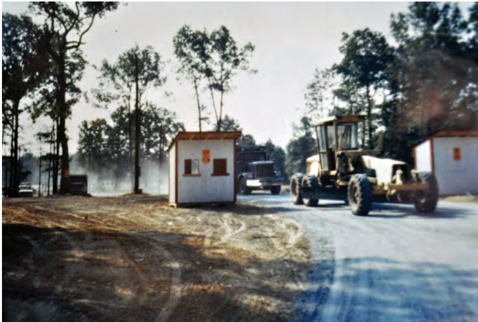
THE CONSTRUCTION OF THE CURRENT FAIRGROUNDS IN 1989
