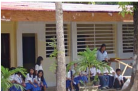
Buenavista Elementary School after repairs were made
