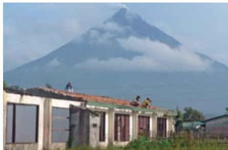
Camalig Elementary School while undergoing repair
