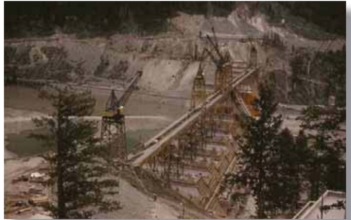
Construction of Libby Dam 1970
