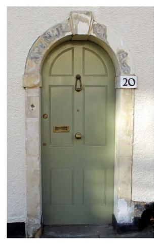
Figure 95: Flush-panel door with limestone surround, Luccombe Hill
