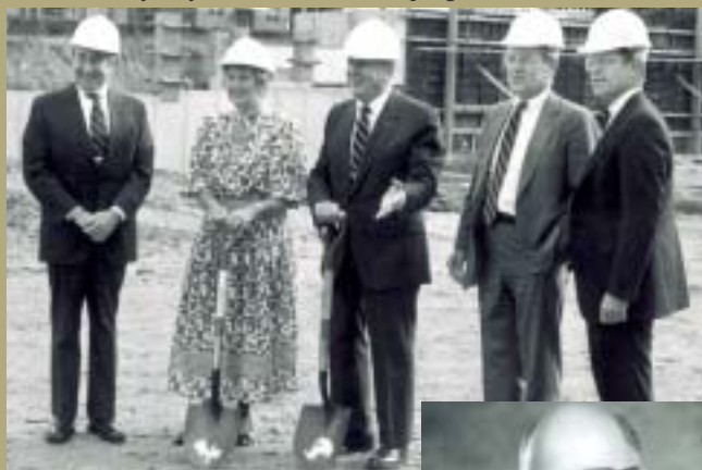
The groundbreaking for the Cancer Center: Dr. Monroe Himmelstein, Helen and Harry Gray, Joe Calhoun, and John Springer
