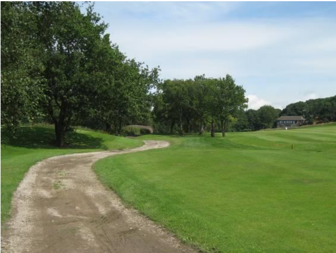
The footpath passes the equipment building (left) with the clubhouse on the right
