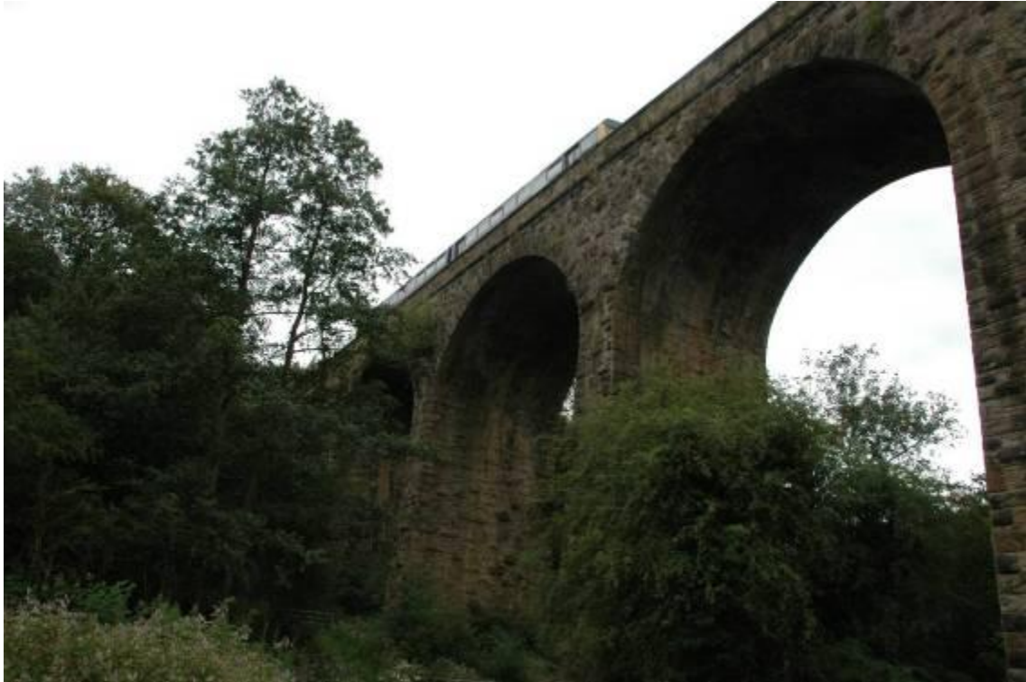
Viaduct over the Goyt
