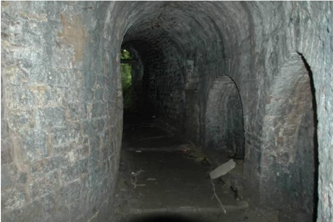
Tunnels under Bottoms Bridge
