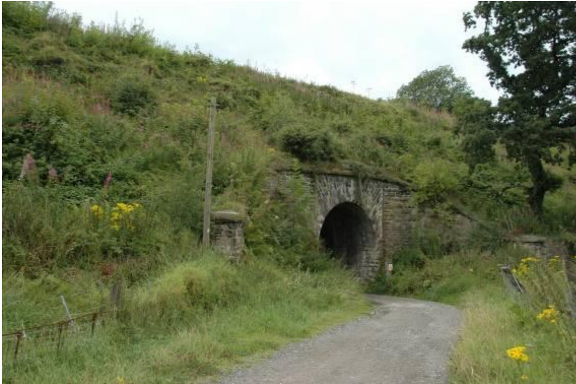
Tunnel at Windybottom Farm
