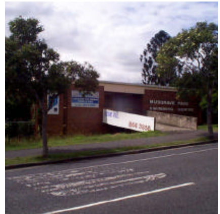
Swimming Pool Entry – Edmondstone St.
