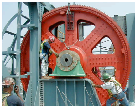
Fig. 7. Sheave Installation
