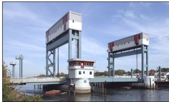
Fig. 2. Present Rte 7 Bridge
