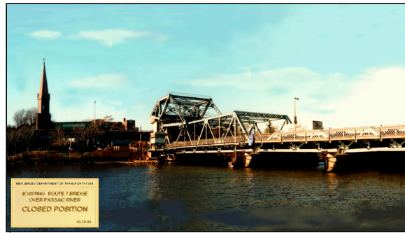
Fig. 1. Former Rte 7 Bridge (Belleville Reformed Church in Background)
