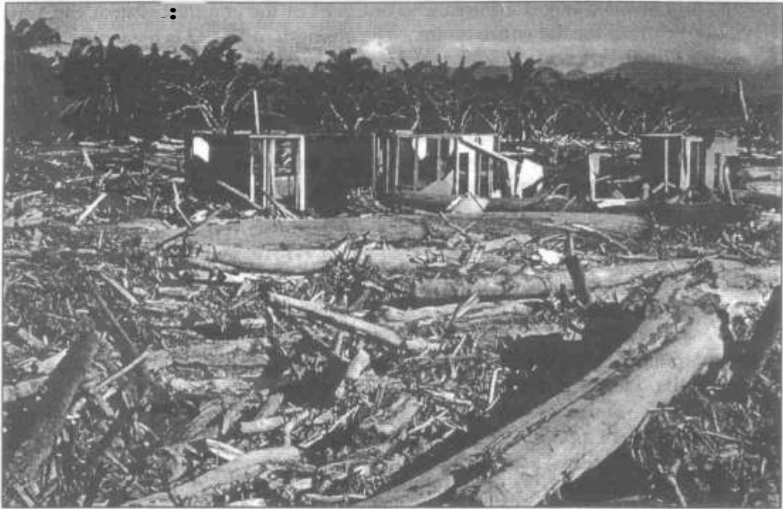
Solomon Islands — damage caused by Tropical Cyclone Namu, May 1986.
