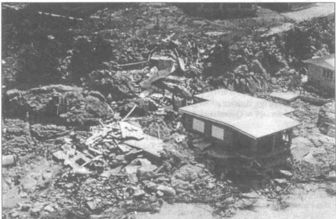
Storm surge damage by Tropical Cyclone Aivu, Wunjunga, Queensland, 1989.
