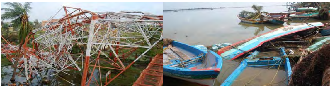
Fig. 2.10.8 Some damage photograph due to the cyclone THANE in Cudallore district Puducherry.
