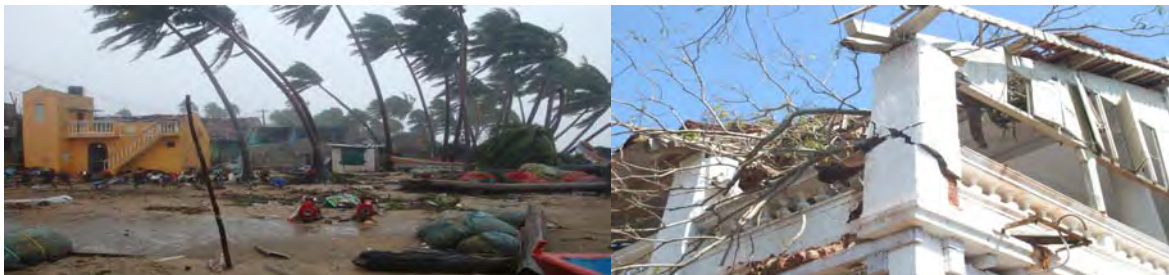
(d) Up rooted trees Pandy Assembly campus and Damaged District Collectorate, Cudallore
