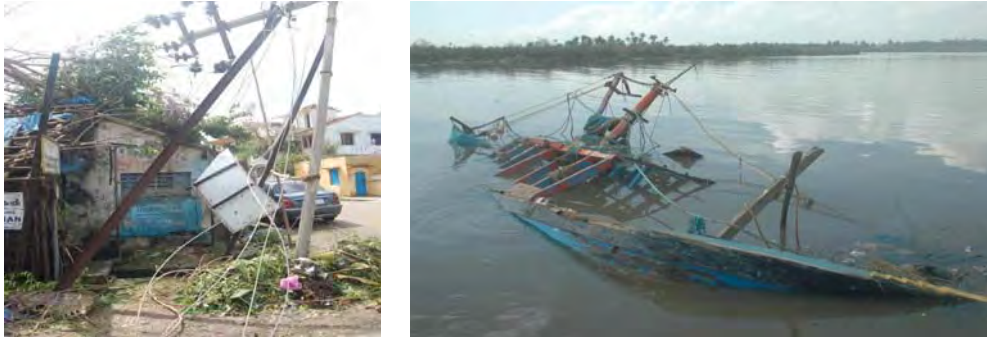
(b) Twisted cell phone tower at Cuddalore and blown up fishing boats at Cudallore
