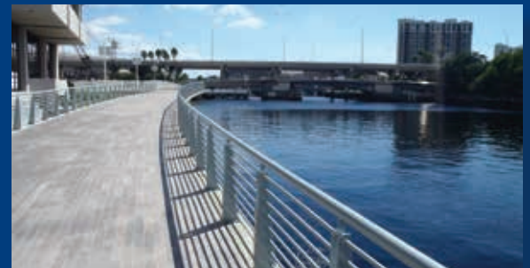
Construction at Tampa's Riverwalk moves to final phases. (Image: Moffatt & Nichol)
