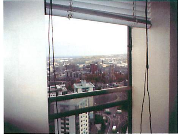
Views of the window wall today
