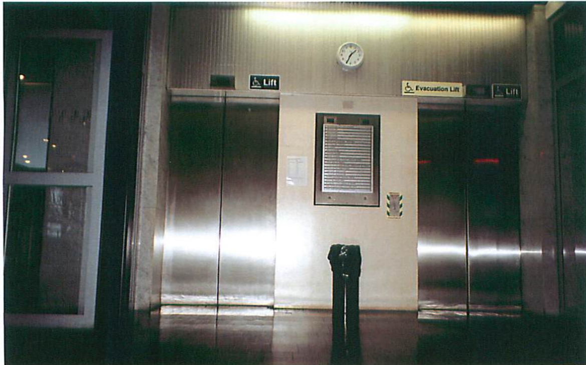
Lift lobby doors and directory
