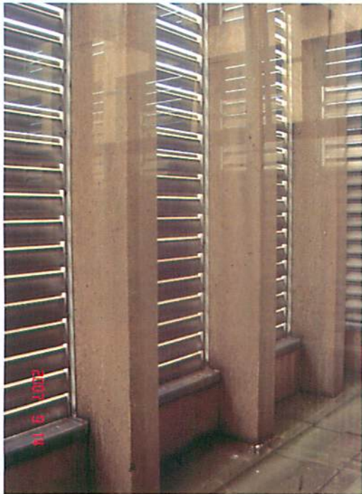
The louvred screen, 19th floor level
