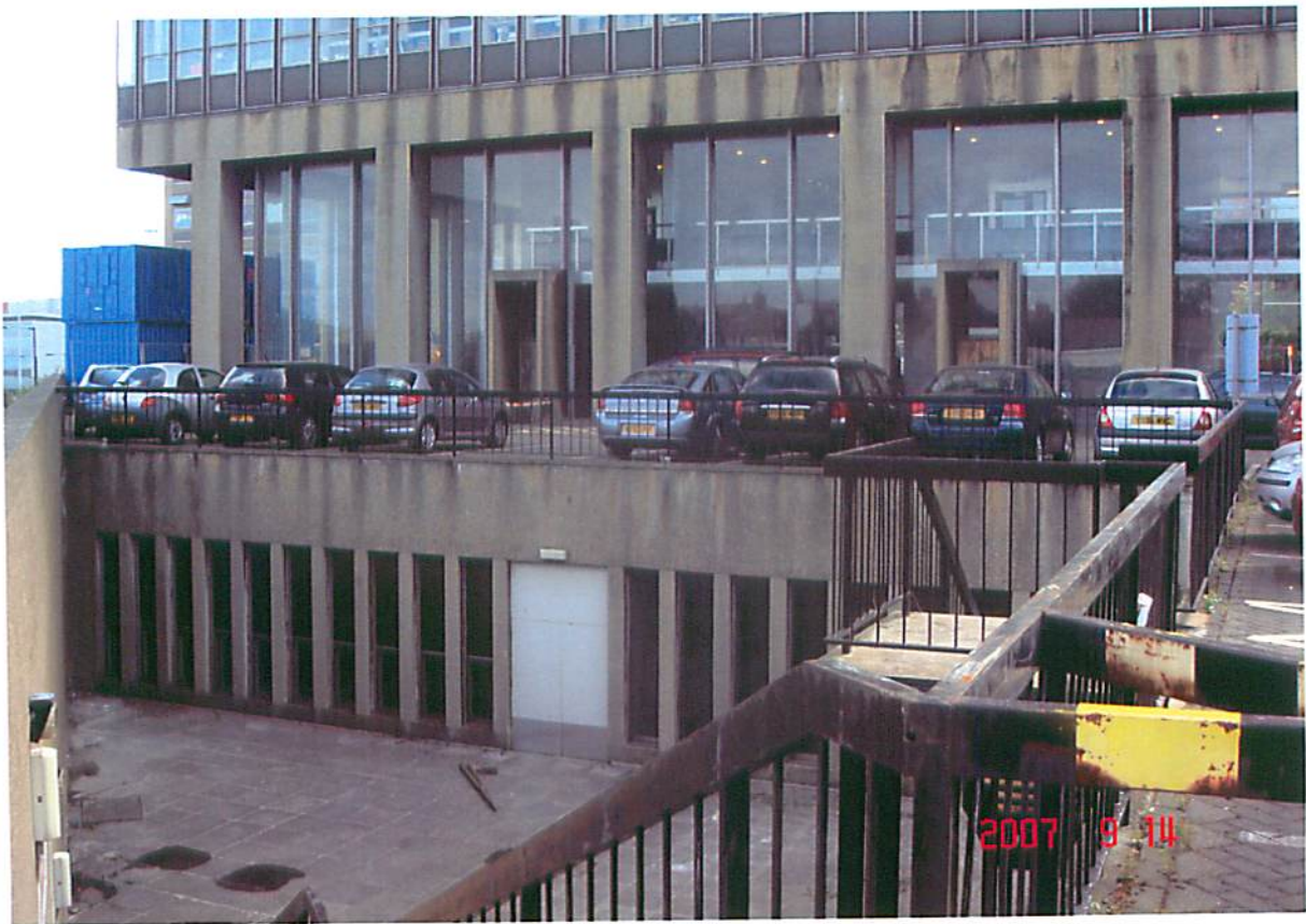
The rear sunken courtyard, and, showing 'sentry box' exits from Tower, and lower level lecture theatres.
