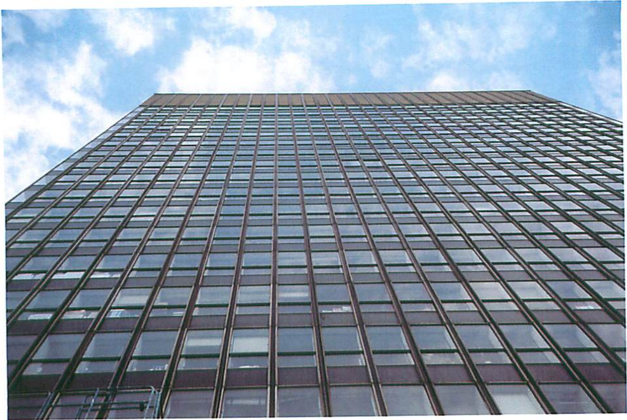
View up the façade showing articulation of flat plane and glass corners
