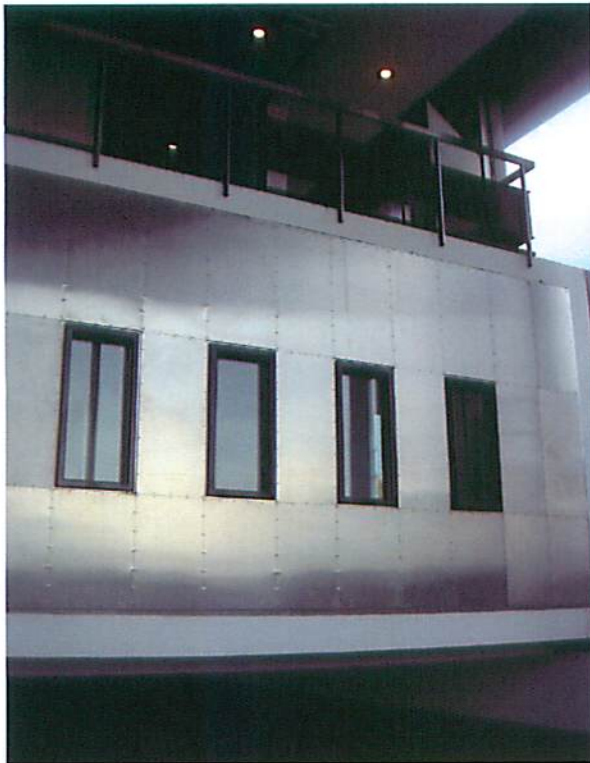
The ground floor escape bridges
