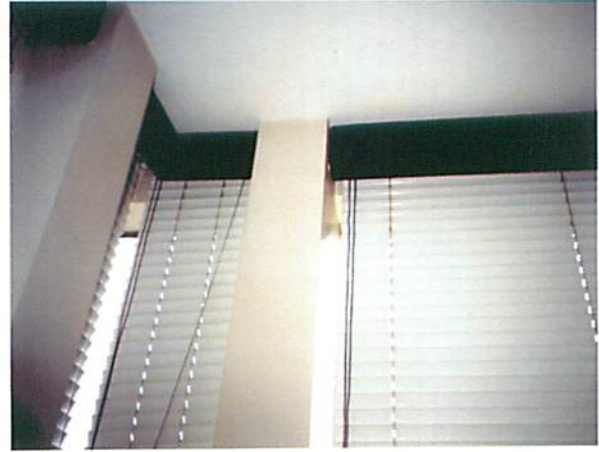
Views of the window wall today
