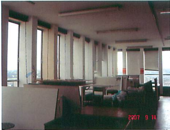
Views of the window wall today
