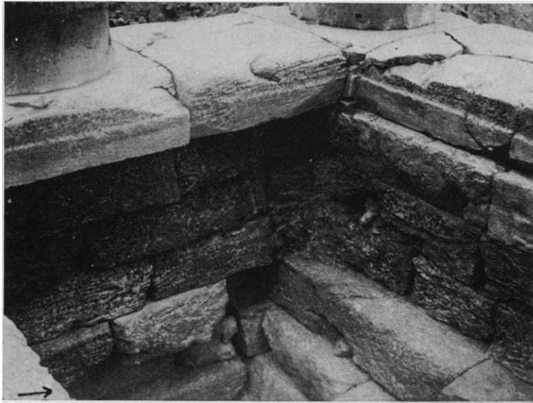
Fig. 14. Foundations below Northwest Corner of Peristyle, from Southeast (Arrow Points to Mason's Mark)
