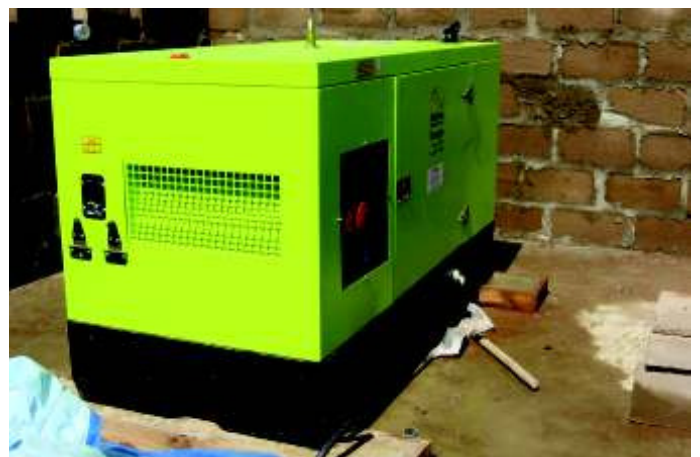
Notstromaggregat
