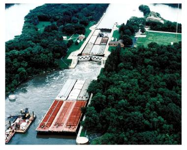
The lock is 110 feet wide by 600 feet long. The maximum lift is 24.5 feet with an average lift lower than 24 feet. It takes an average of 15 minutes to fill the lock chamber; 10 minutes to empty it.
