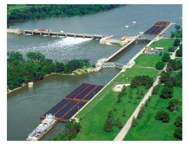
The dam consists of an arch dam section, a fixed spillway section, nine Tainter gates (60 feet wide by 17 feet high), 18 plugged headgates, and a 500-foot-long earthfill section with steel sheet pile cut-off wall connecting the headgate section to the Illinois and Michigan Canal embankment.
