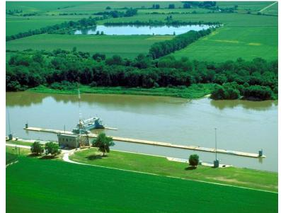
feet wide by 14.92 feet high, with a .25-foot gap between wickets. From 1987-1991, a major rehabilitation changed the physical components of the dam and operating procedures by replacing 26 of the original 135 wickets with a single 84-foot long submersible Tainter gate adjacent to the lock wall.
