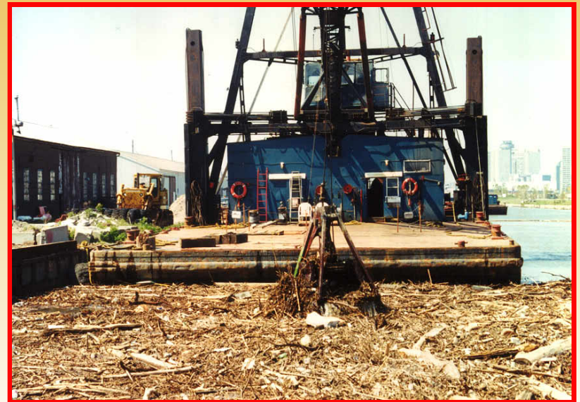
Derrick THC 50 removing debris.
