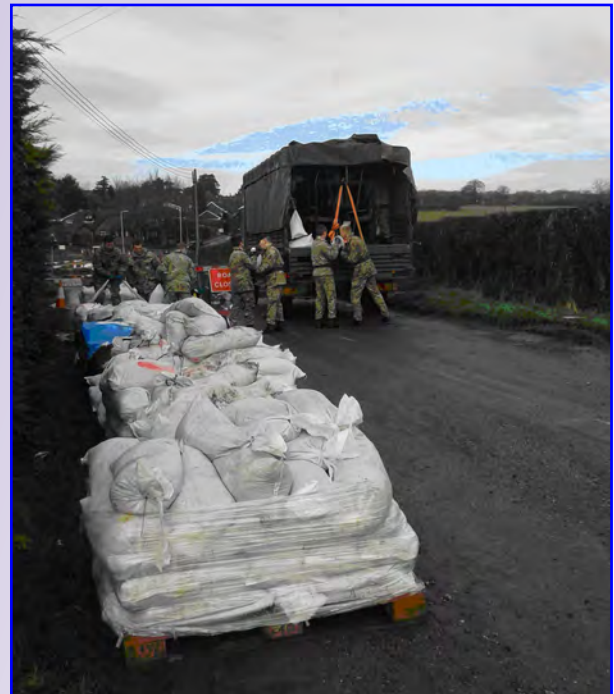
Loading sand bags onto the MAN SV for flood defence building
