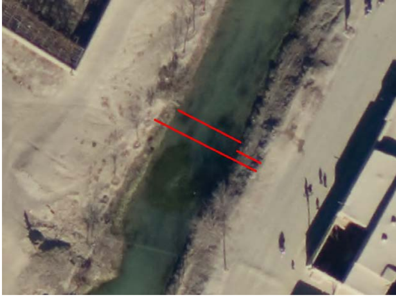
Figure 4. Representative Section of Sluice Channel: Nov 2010. Red lines are channel width, sediment width, and exposed sideslope width resp.
