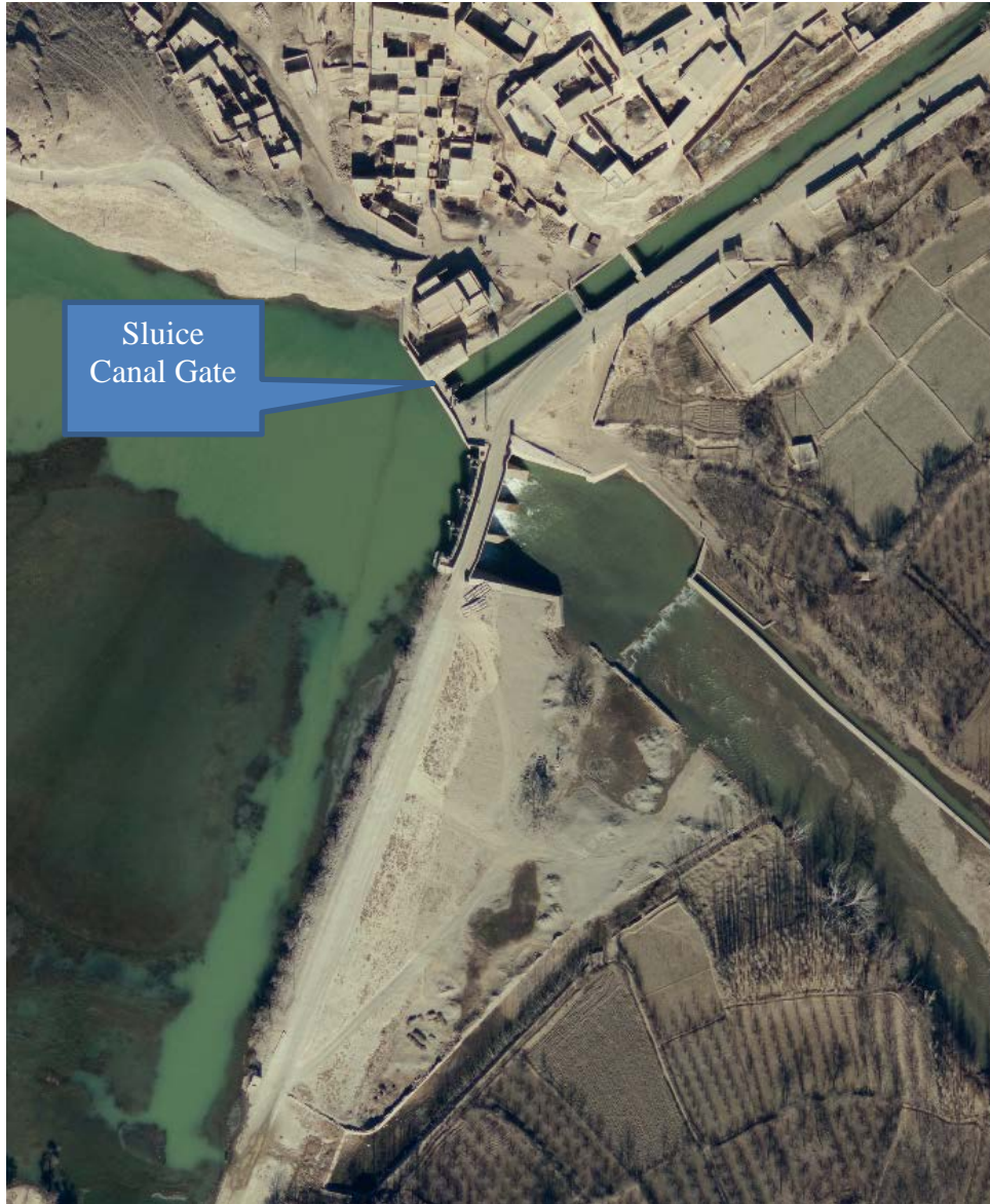
Figure 1. The Chak E Dam in Wardak Province (Nov 2008)
