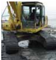
Even in extreme tidal conditions our heavy duty mats provide a strong stable base.
