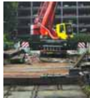
Heavy duty crane access mats
