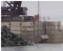
Our Heavy duty platform protection mats.
