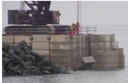
Our Heavy duty platform protection mats.
