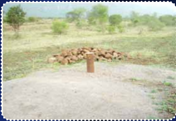
1. Drilled bore hole at mbagave community under mkhiweni inkhundla
