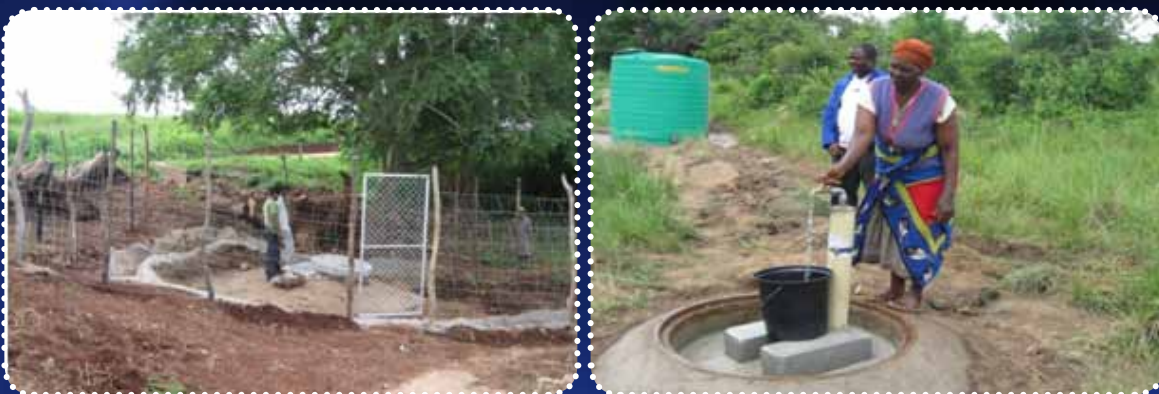
13. Completed spring protection maphungwane community
