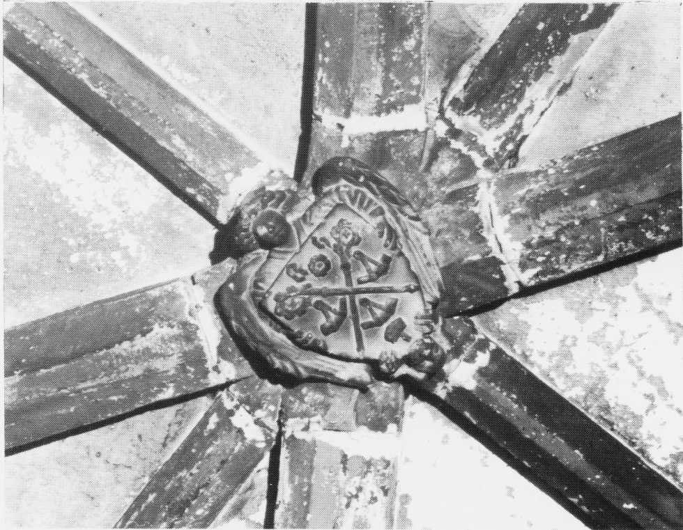
Fig. 5. Mauchline Castle, first-floor rib-vaulted ceiling, detail of N boss 1977.
