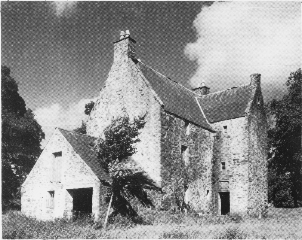
Fig. 1. Barscobe House, from SW 1971.
