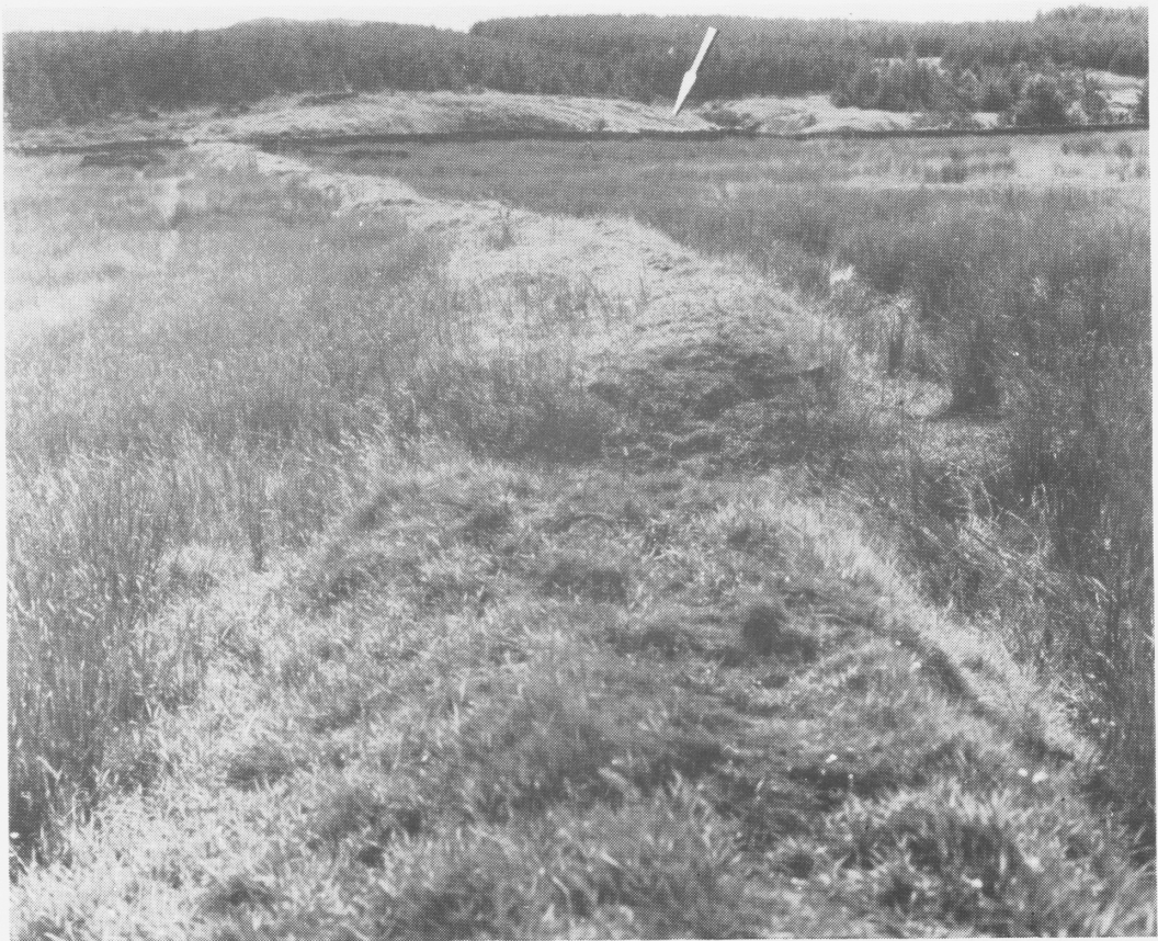
Fig. 2. A view E. along the Deil's Dyke in the W sector. Note the angular join and the gap (foreground). The arrow indicates the probable position of the W end of the C sector.
