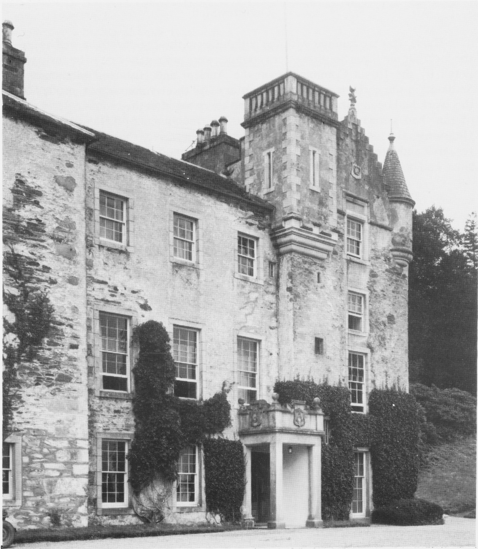
Fig. 2. Cassencary House, central block from NW 1958.
