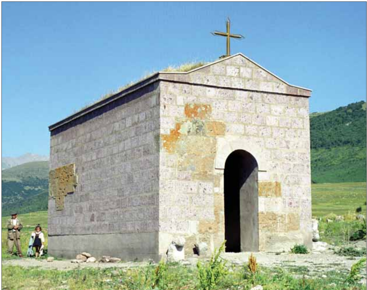
Merena Village, Javakhk. Kotratz Church from the north-west (1988) and after its self-willed "restoration" (2001)
