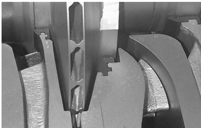
Figure 18. Photograph Illustrating the Use of Tape to Determine Radial Seal Clearance in the Upper Half of the Compressor.
