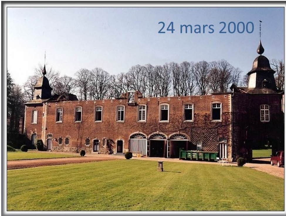
View from the South Wing after the fire
