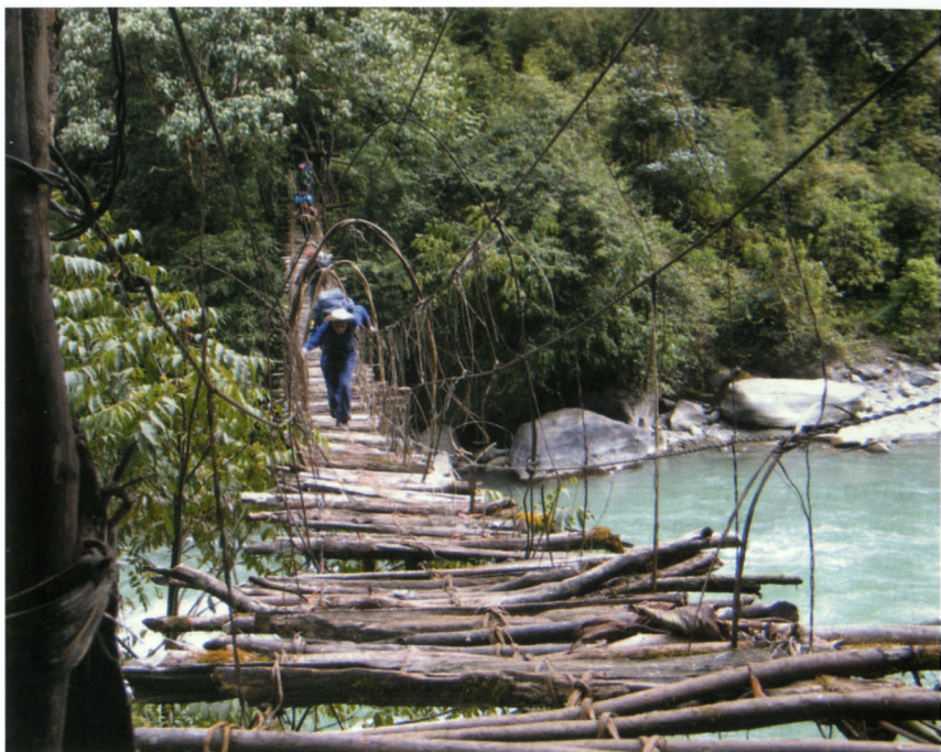
153. Bamboo suspension bridge on the Old Pilgrimage Route to Takpa Siri. (Harish Kapadia collection)
