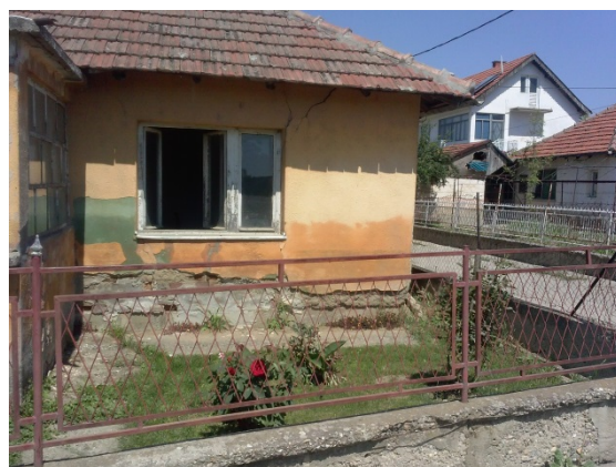
Figure 1-32. Smed. Palanka, after the floods water receded
