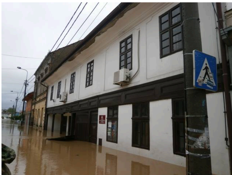
Figure 1-37. Flood Damages in Obrenovac:
