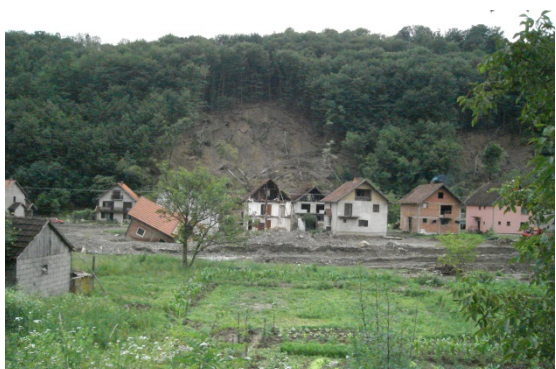
Figure 1-33. Krupanj, effects of landslides and flooding
