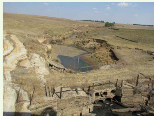
Figure 42: Looking downstream Vaal crossing
