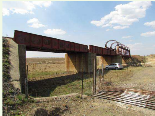
Figure 40: View of railway cross-section
