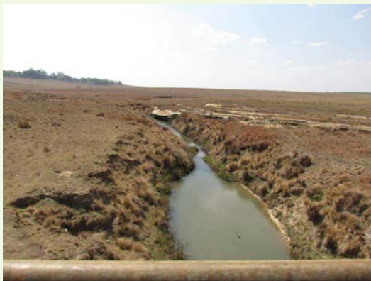
Figure 41: Looking upstream Vaal crossing
