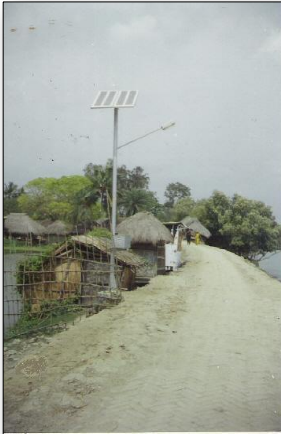
Solar street lighting.
