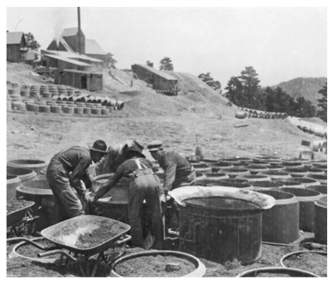
Figure 2. Workers fabricating steel-reinforced concrete gravity pipeline sections at one of the work sites (perhaps Magnolia work camp) established during the project. Photo: Carnegie Branch Library for Local History, Boulder, Colorado, *Boulder Daily Camera* Collection.
