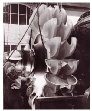
Figure 7. A worker heating the hub of the new water wheel, June 1959. Photo: Betasso Water Treatment Collection.
