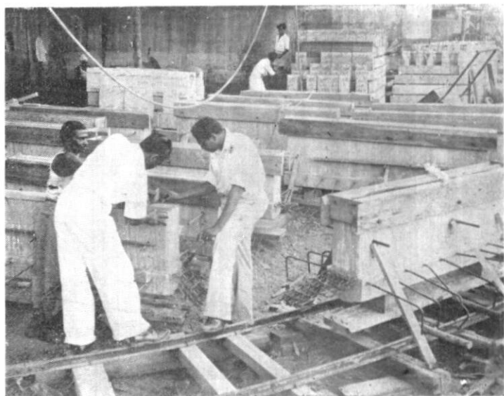
Fig. XI. Checking R.C. rollers (precast).
