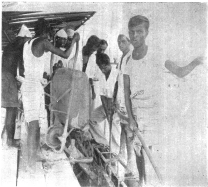
Fig. XII. Concreting of a parapet beam.
