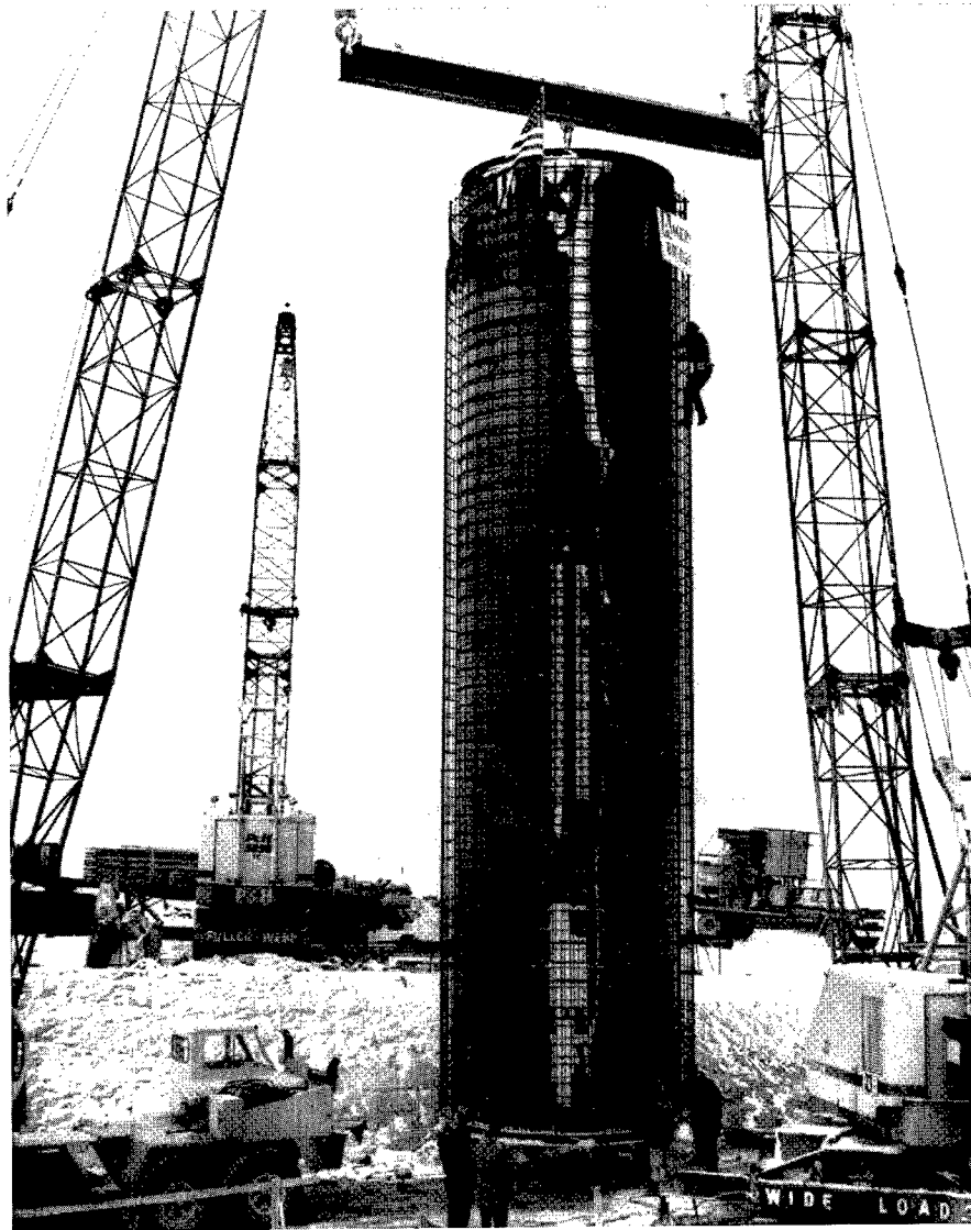
Workers from U. S. Steel's American Bridge Division put the finishing touches on the last of more than 100 silo liners it installed in Minuteman launch facilities around Malmstrom AFB, Montana.
