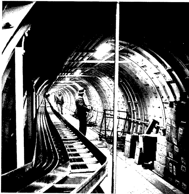
In this 1960 photograph, work on the main tunnel of the Titan I launch complex at Vandenberg AFB nears completion. Forty feet beneath the surface, the tunnel connected the control center to the missile silos.
