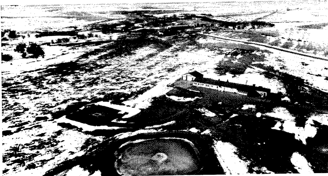
An aerial view of Minuteman launch control facility D-1. The building in the center of the photograph is the launch control facility support building.
