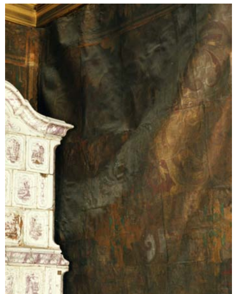
Fig. 2. Gilt leather curled and bulged. The soiling of the surface made interpretation of the ornaments and colours difficult. State of preservation before conservation.
