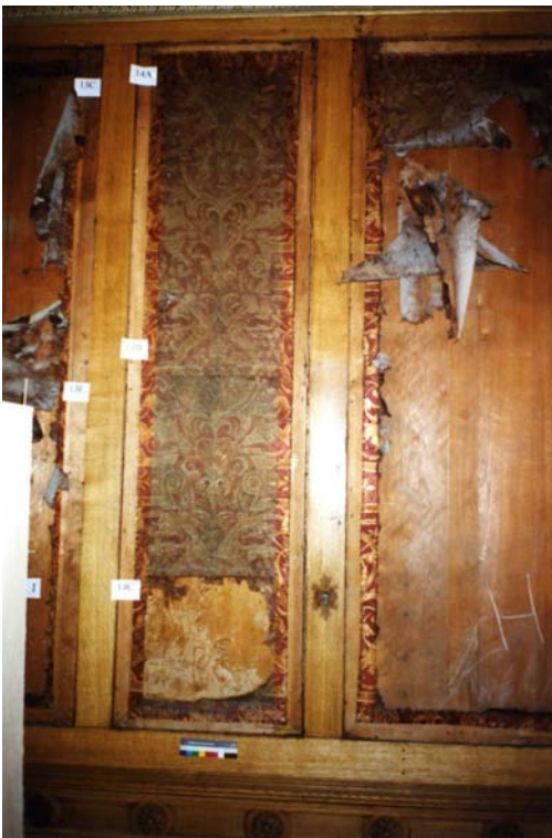
Fig. 1. Original gilt leather wall hangings decorating the Callendar House in Scotland. The original way of mounting the leather on wooden panels placed on the walls is shown.
