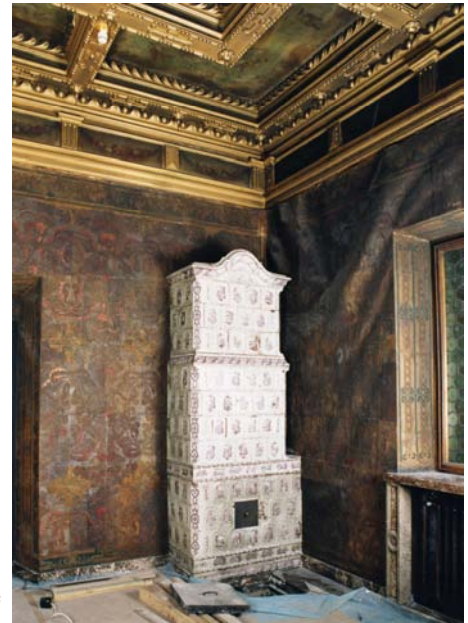
Fig. 1. Gilt leather wall hangings decorating the Antechamber of the 'Kurza Stopa'. State of preservation before conservation.
