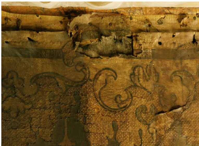
Fig. 3. Areas of damage to the edges of leather and canvas caused by faulty fixing of the gilt leather. State after surface cleaning.
