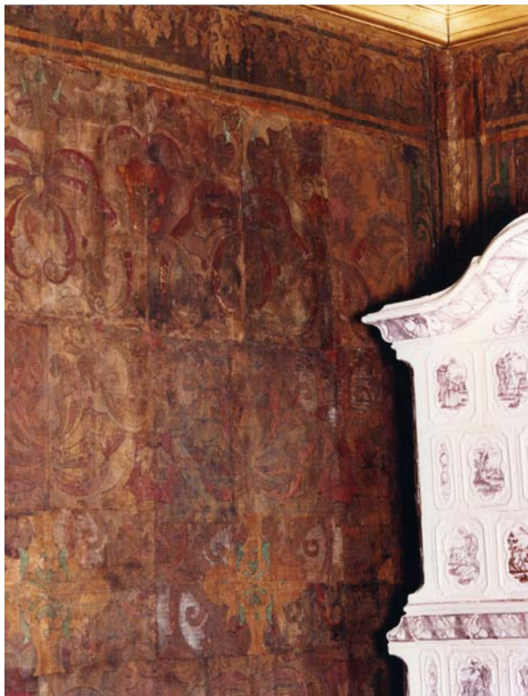
Fig. 8. Gilt leather stretched and flattened. The state after the completion of the conservation works.
