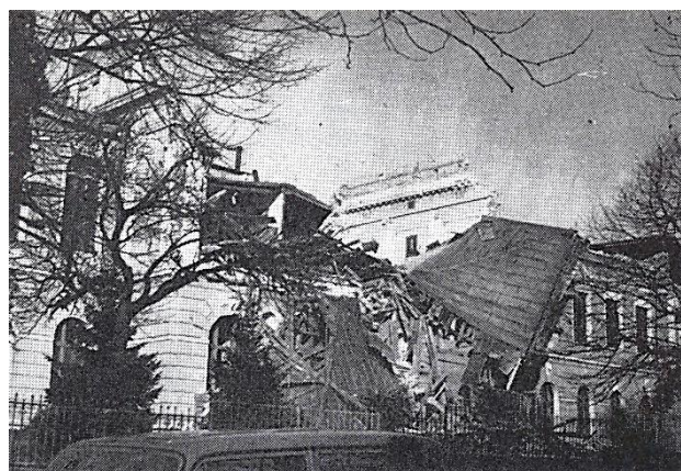
Fig. 7. Economic College in Svishtov (N Bulgaria) ruined by 1977 Vrancea earthquake (Mw 7.5) [2]
