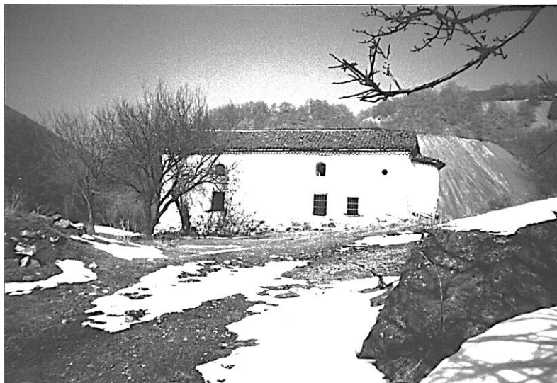
Fig. 8. The Seslavtsi monastery (W Bulgaria) that was damaged by a number of man-made earthquakes, and seemingly by natural quakes as well
