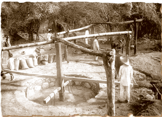
Instalación para trituración de grava, con tracción animal. © Wicks, S. Robert & Harrison H. Roland, Buried Cities, Forgotten Gods. William Niven's life of discovery and revolution in Mexico and the American Southwest , Texas Tech University Press, 1999.
