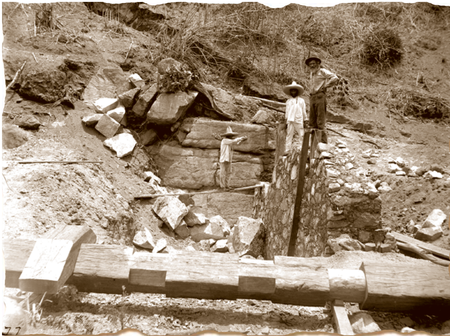
Foto 4: Construcción de canal de agua y de una rueda hidráulica. Placeres del Oro. © Wicks, S. Robert & Harrison H. Roland, Buried Cities, Forgotten Gods. William Niven's life of discovery and revolution in Mexico and the American Southwest , Texas Tech University Press, 1999.
