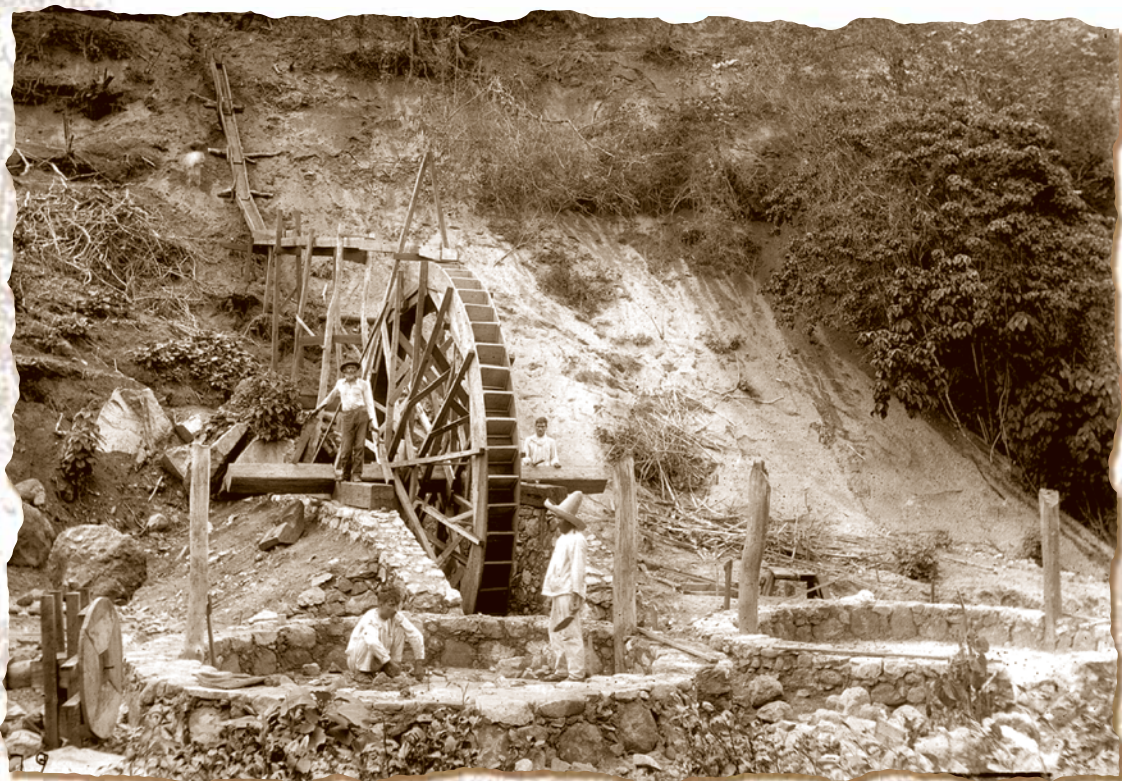
Foto 6: Instalación de canales y rueda hidráulica para lavar oro. Placeres del Oro. © Wicks, S. Robert & Harrison H. Roland, Buried Cities, Forgotten Gods. William Niven's life of discovery and revolution in Mexico and the American Southwest , Texas Tech University Press, 1999.
