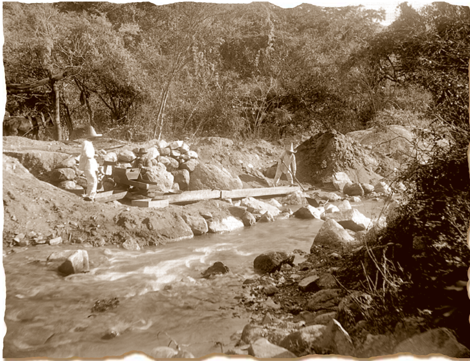
Foto 2: Extracción de oro, a partir de cajones en los que se lava graba, Placeres del Oro. © Wicks, S. Robert & Harrison H. Roland, Buried Cities, Forgotten Gods. William Niven's life of discovery and revolution in Mexico and the American Southwest , Texas Tech University Press, 1999.
