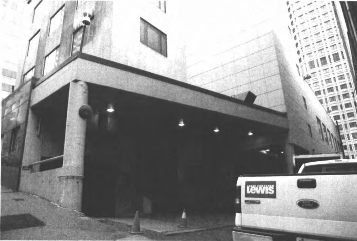
5 of 22: 2011 view of north and west facades. Source: Artifacts Consulting, Inc.
