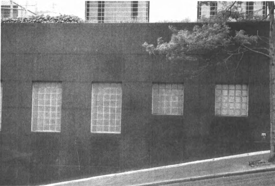
9 of 22: 2011 detail of original glass block windows in south facade. Source: Artifacts Consulting, Inc.
