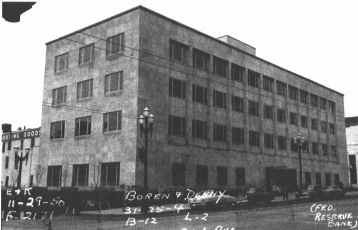
November 29, 1950 view of south and east facades. Source: Puget Sound Regional Archives.
