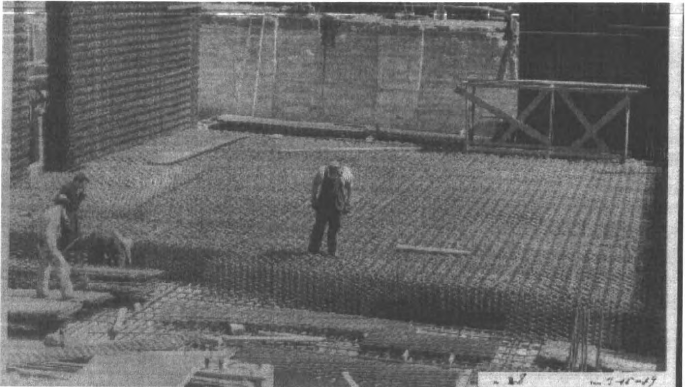
1949 view of lower vault construction. Source: Federal Reserve Bank Archives.
