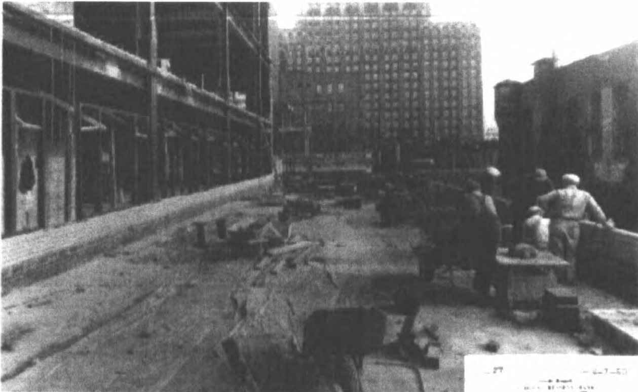
1950 view looking south across 2nd floor roof. Note start of brick courses and window framing. Source: Federal Reserve Bank Archives.
