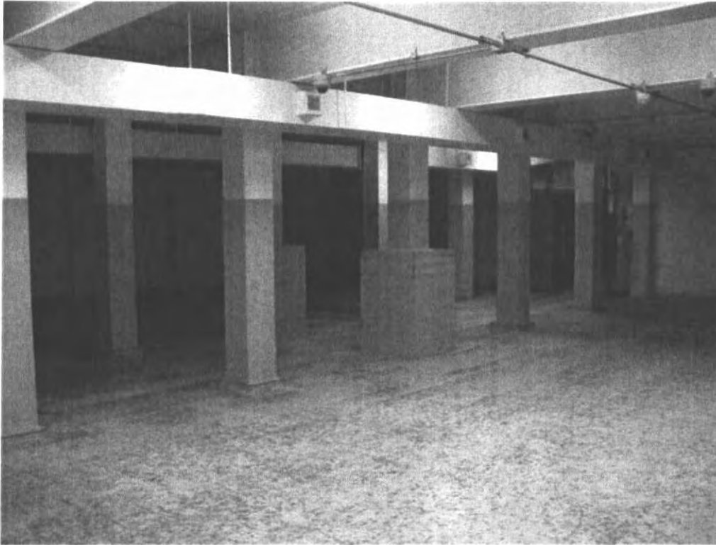
17 of 22: 2008 interior view of lower vault. Photo by Art Skolnik.
