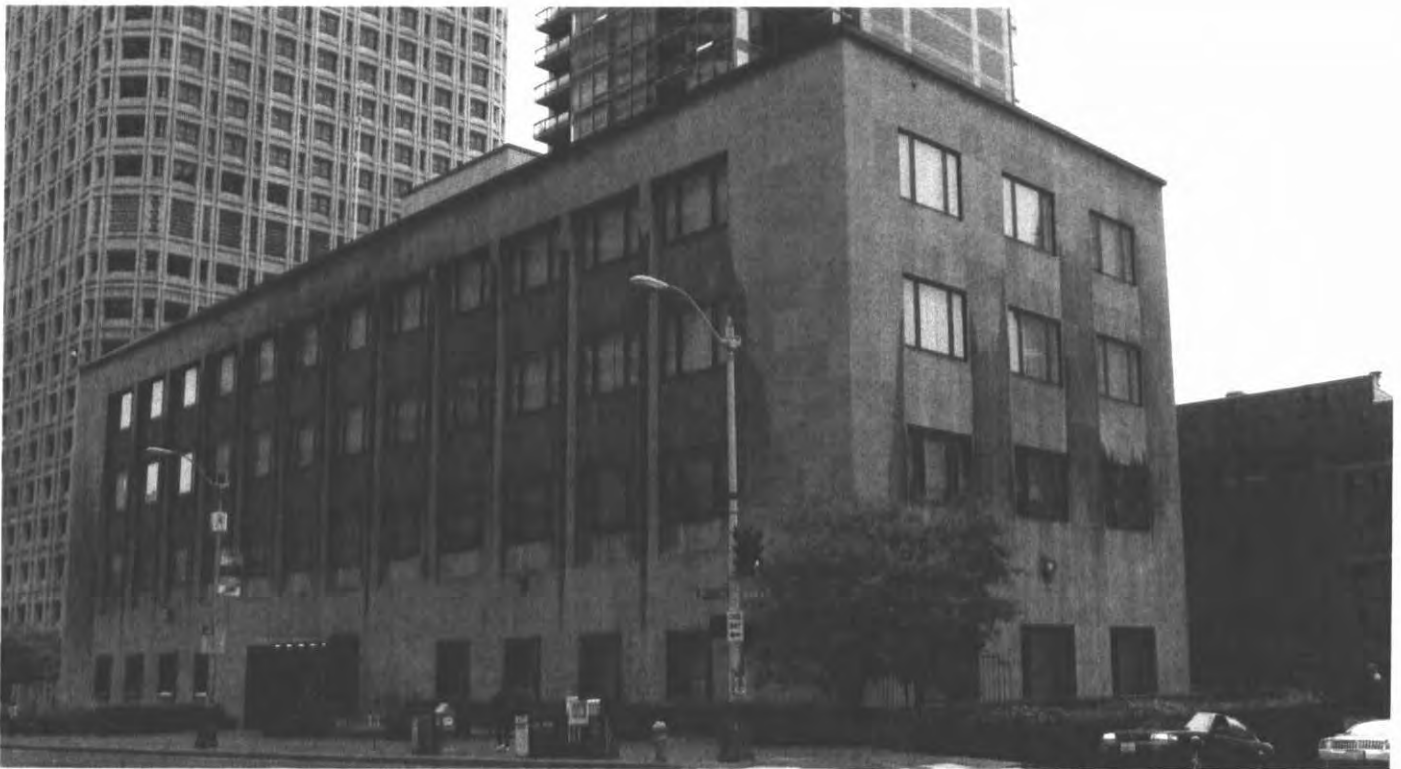
2 of 22: 2011 view of east and north facades. Source: Artifacts Consulting, Inc.
