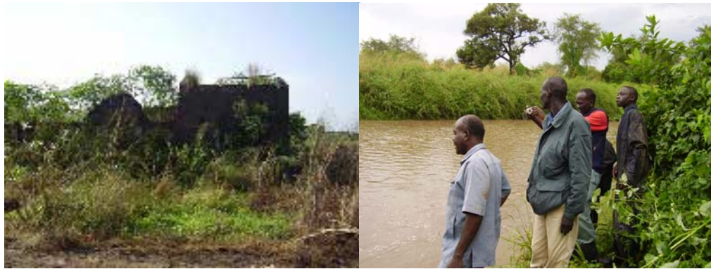
Destroyed school building; and Diem Mansour-Chali road with seasonal river flooded ( mission got stranded overnight because of flash floods )
