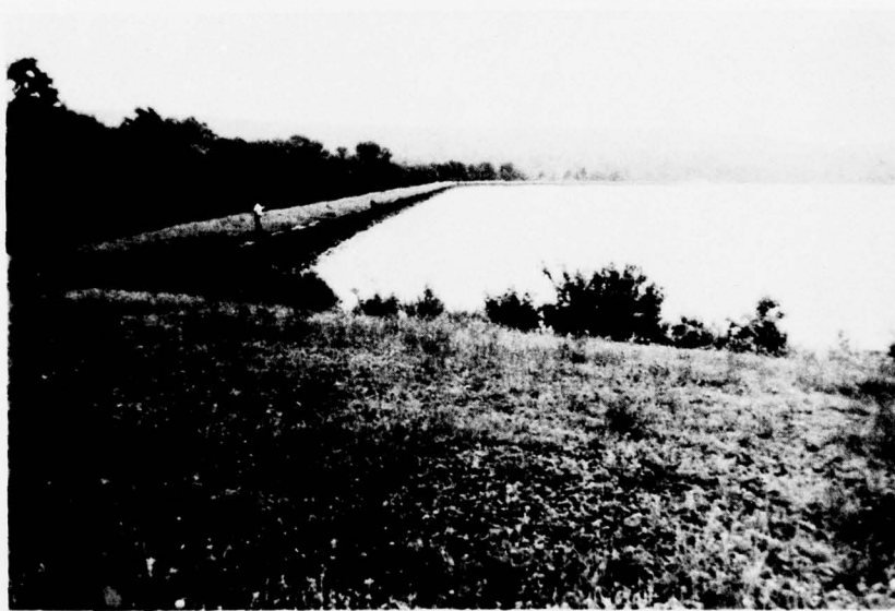
B. Embankment — View from Auxiliary Spillway at Left Abutment
