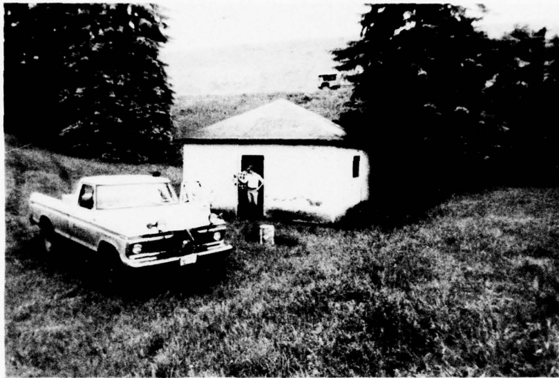
I. Valve House — Embankment in Background
