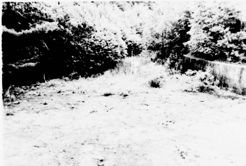
H. Auxiliary Spillway Channel
