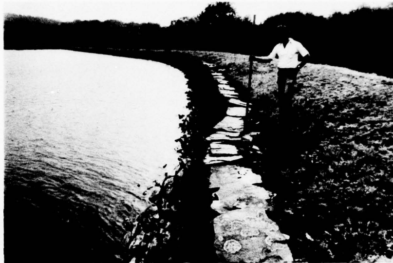
C. Riprap on Upstream Slope
