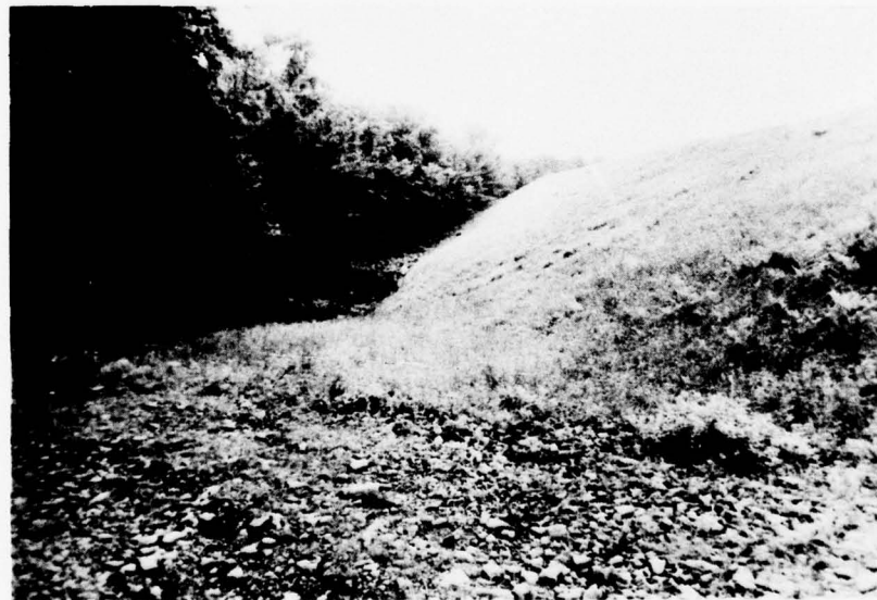
D. Embankment and Wet Area Near Left Abutment
