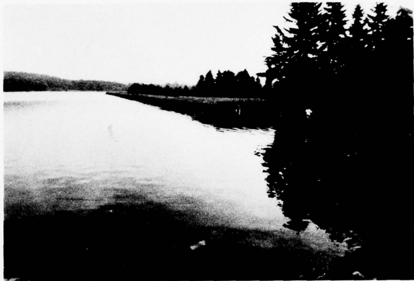
A. Embankment and Main Spillway View from Right Abutment
