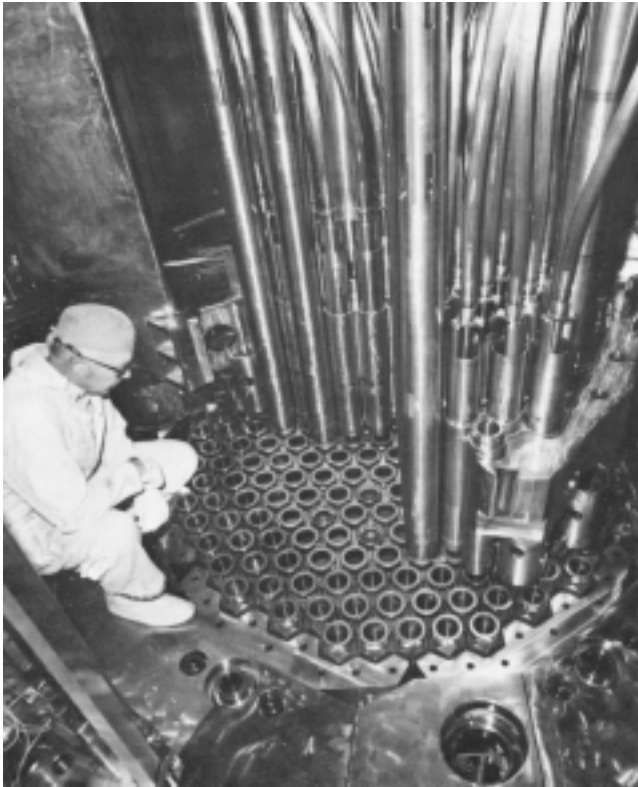
The FFTF fuel assembly grid (below) with reactor operating equipment (above). Pelletized fuel of mixed uranium-plutonium oxide is stacked in a 3-foot column inside stainless steel tubes to form fuel pins, which are arranged in 217-pin assemblies for insertion into the core. Samples of nuclear fuel and other breeder reactor materials are placed in the core for testing.
