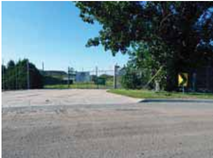
HOLMESGLEN TAFE INDUSTRIAL SKILLS SITE
