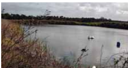
CONSTRUCTED DAM CLOSE TO MORDIALLOC SETTLEMENT CREEK
