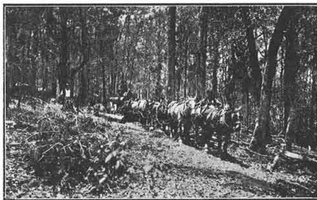
HAULING TIMBER IN TYPICAL FOREST COUNTRY, RAVENSHOE DISTRICT, NORTHERN QUEENSLAND.
