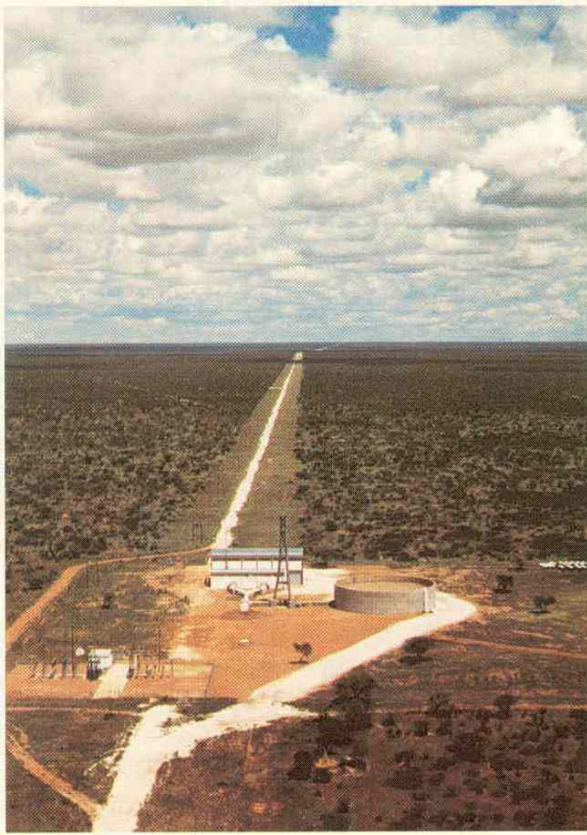
Booster pump station and buried pipeline
