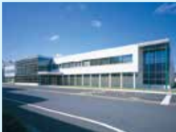
Internal broaches factory
