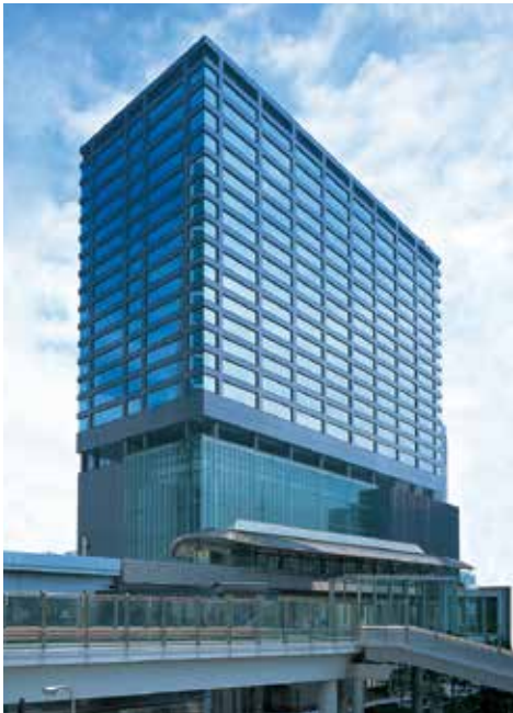
Tokyo Head Office, Eastern Japan Branch Office Shiodome Sumitomo Bldg.
