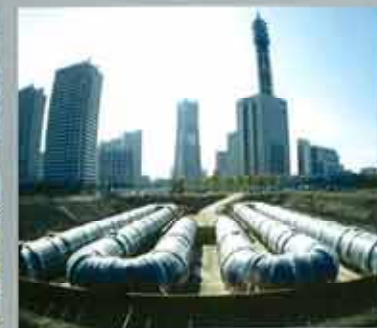
災害用地下水タンク (50万人分の飲料水3日分供給可能) Emergency underground water tanks (Storage of a three-day supply of drinking water for a half million people)
