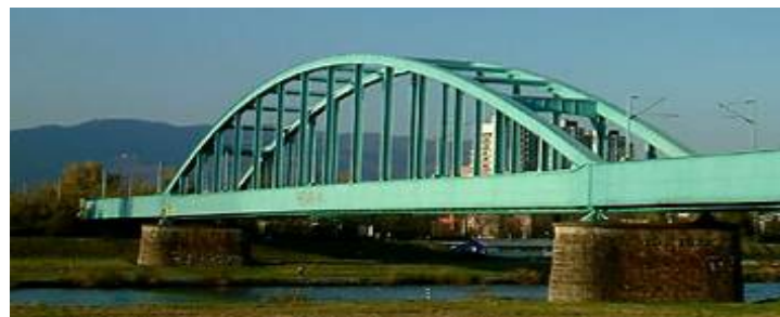
Figure 15 : View of the Railway Bridge
