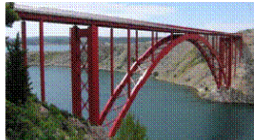
Figure 9 : Construction Maslenica Bridge (top), and view of new bridge (bottom)
