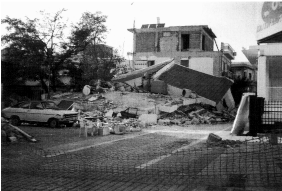
Fig. 10. A brick masonry and reinforced concrete slab construction with almost nonexistent supporting columns that collapsed in Ano Liosia.
