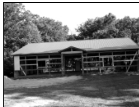
The Clubhouse is under construction.
