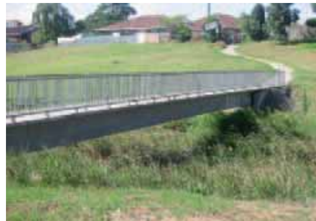
Figure 40: Footbridge across Kororoit Creek
