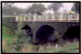
Historic bluestone bridge
