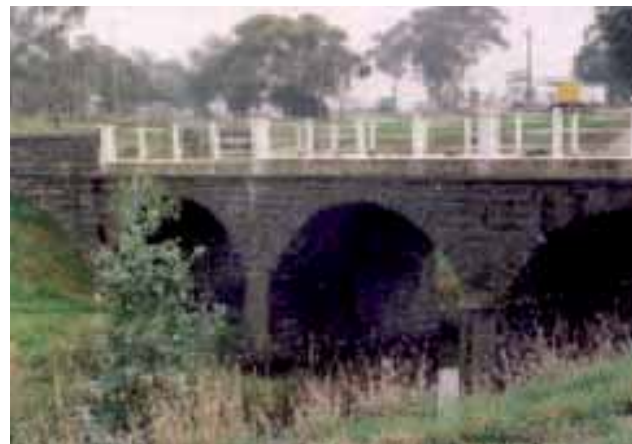
Figure 43: Old Geelong Road Bluestone Bridge (Princes Highway can be seen Beyond)
