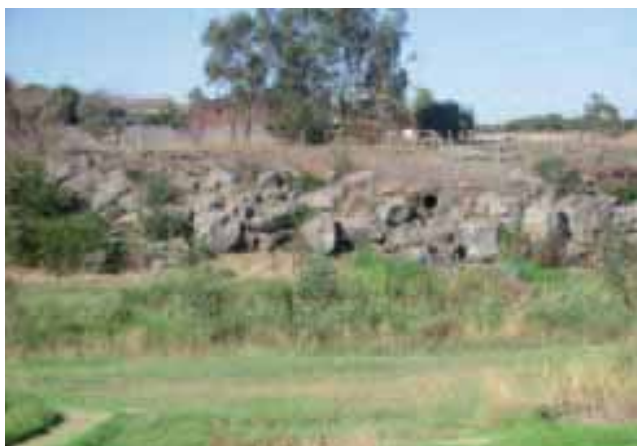
Figure 31: Rock Escarpments and Drain Outlet in Deer Park
