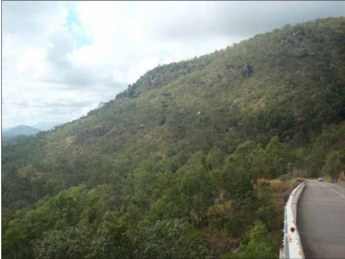
Photograph 17: View looking down Hervey Range Road. Note steep escarpment above road with large bedrock outcrops (potential rock roll source).
