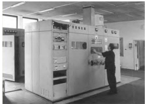
100 kW SW "Tesla" transmitters near Warsaw were shortly tested for jamming of the RFE Polish programs in December of 1970.
