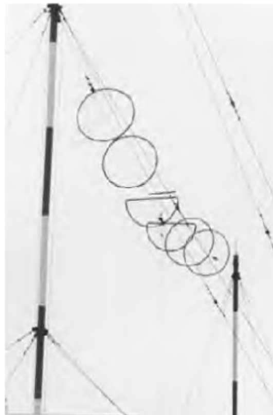
Standard multi-wire broadband "VGDSH" type dipole, used for ground wave jamming in the USSR
