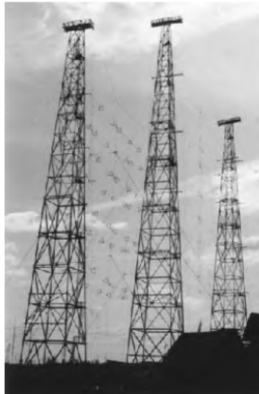
Vertical curtain array SW antennas, used for the long-distance sky wave jamming
