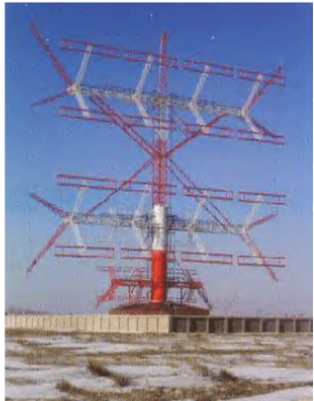
Sky-wave jammer near Kashi in Xinjian province, western China (39N20/75E46): one of 13 rotatable Thales ALLISS antennas with 500 kW Thales TSW2500 transmitters
